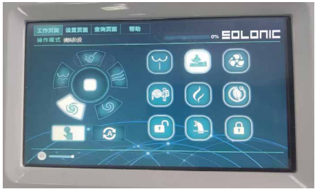
After the installation is completed, perform a manual defecation process
